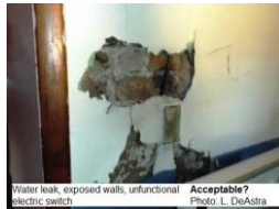
Water leak, exposed walls, unfunctional electric switch
