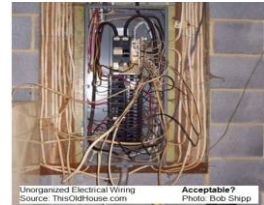
Unorganized Electrical Wiring Source: ThisOldHouse.com
